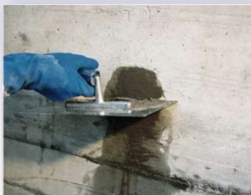
Level off surface.
