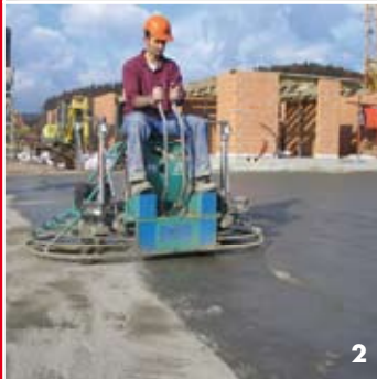
2 Working the powder into the surface by machine or hand trowel.
