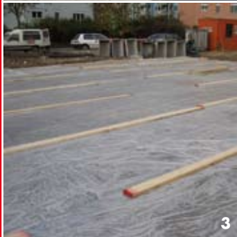
3 Curing and protection for 5 days against evaporation by sun and wind.
