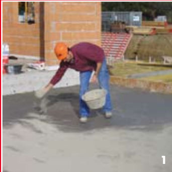
1 VANDEX SUPER dry-sprinkled as powder immediately after initial setting of concrete.
