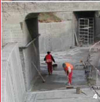
4 Alternatively apply VANDEX SUPER as a slurry .
