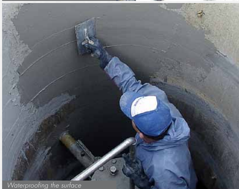
Sealing of leaking points
