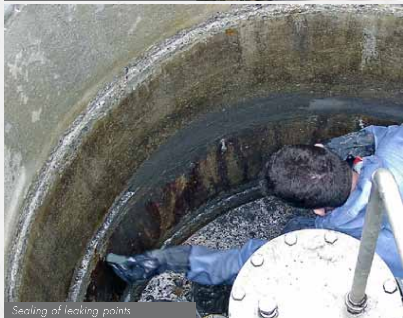
Substrate preparation
