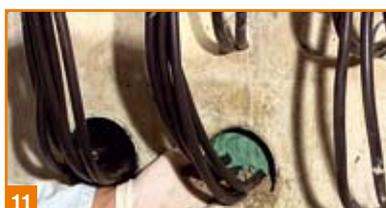
Apply mortar in the remaining 50mm of the duct. Start at the bottom between the cables.
