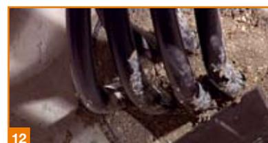
Smoothen the surface of the mortar by using a putty knife and some water.
