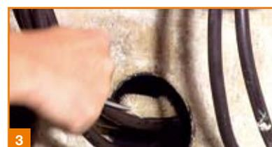
Duct to be cleaned using a brush and cleaning pad. Cleaning with water afterwards is optional, STOPAQ® 2100 Aquastop adheres to wet and dry surfaces. Adhesion can be improved when cables and duct are pre-applied with 2100 Aquastop.
