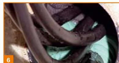
Lift the cables and apply STOPAQ® 2100 Aquastop with an appropriate application gun around the cables. Use the flexible nozzle to fill 100mm of the duct without air enclosures. Apply from the rear of the duct to the front.
